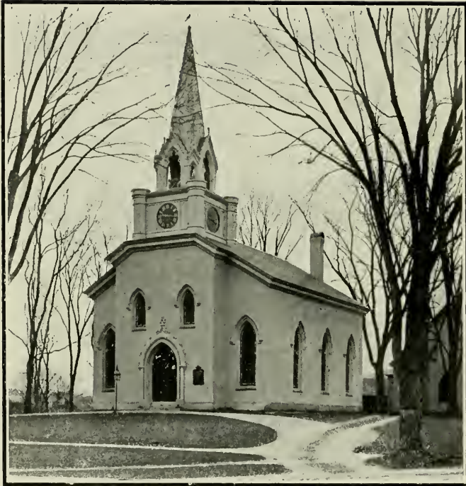
SOUTH PARISH CHURCH, 1905
